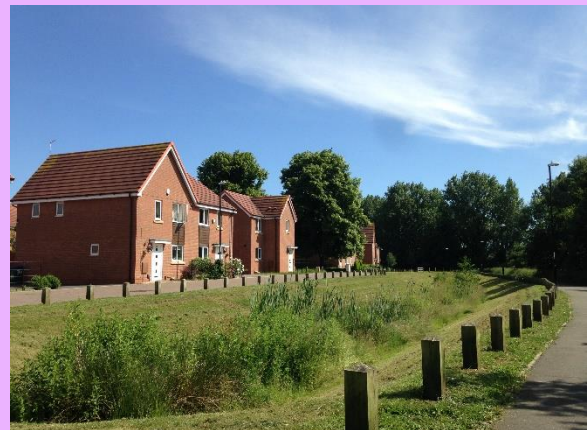
An attenuation basin (left) and swale (right). Part of a SuDS scheme on a redeveloped housing estate in Wood End, Coventry
