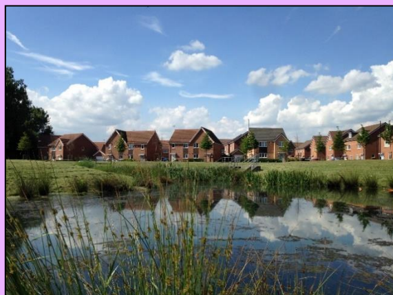
An attenuation basin (left) and swale (right). Part of a SuDS scheme on a redeveloped housing estate in Wood End, Coventry
