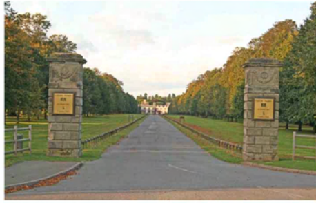
Study areas C5 and C6 form the setting of the Combe Abbey estate.
