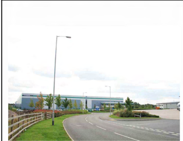
The Prologis Park development at Keresley is a largescale commercial development on a former colliery site. It is prominent in many local views. Around Keresley there is a variety of 'urban fringe' landuse and declining farmland. However it is considered that settlement sprawl needs to be contained in this locality and that the Green Belt should be protected and enhanced.
