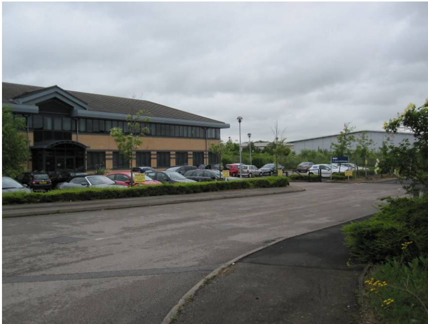
Typical office and warehouse buildings at Cross Point Business Park
