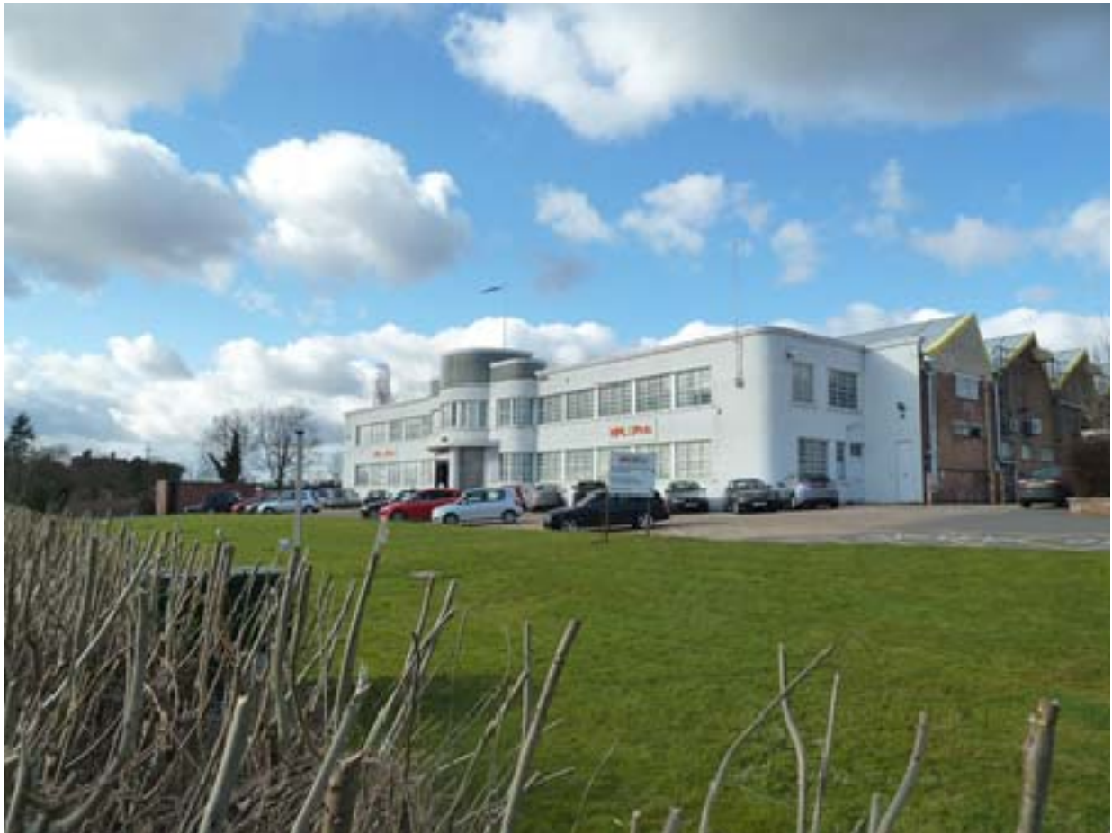
1930s Art Deco building at the Windmill Industrial Estate
