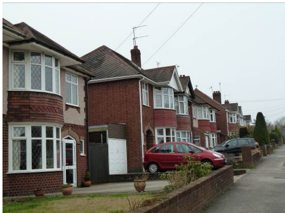
Typical residential properties in Brayford Avenue
