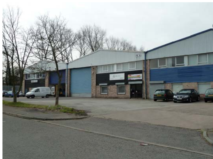
Typical industrial units at Binns Close
