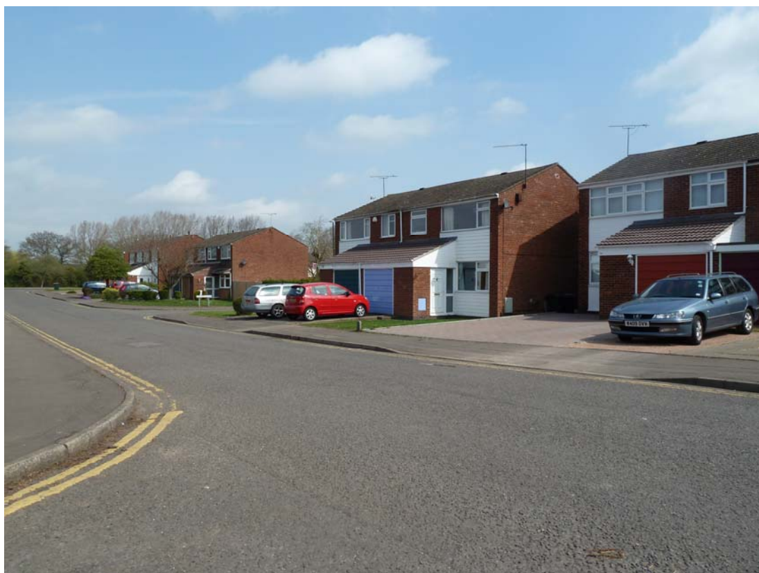
Typical semi-detached houses on Blandford Avenue
