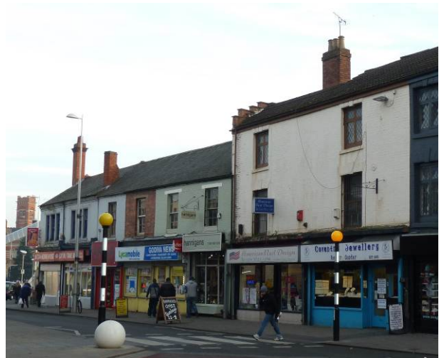
Modern shop fronts on historic buildings and projecting signs and A-boards creating clutter
