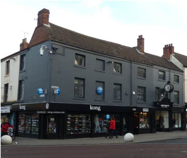
Intrusive signage and CCTV camera at no. 18 Burges
