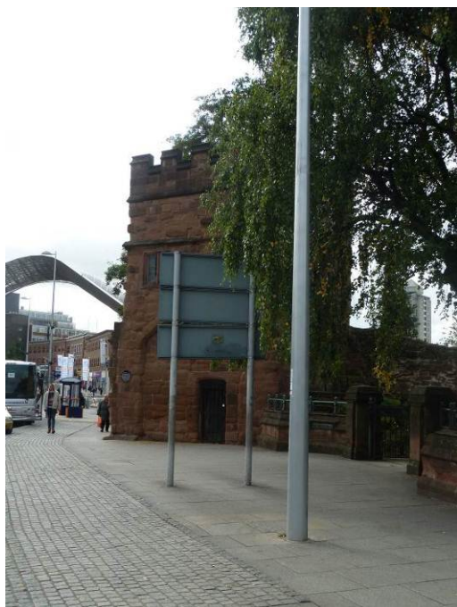
Poorly positioned road signs, lamp posts etc. obscure view of Swanswell Gate on Hales Street
