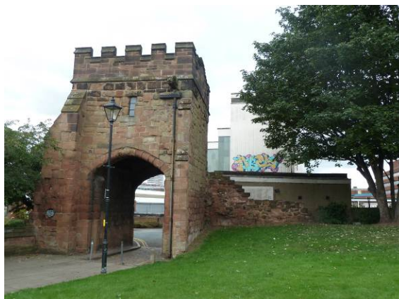
Graffiti on building adjacent to Cook Street Gate
