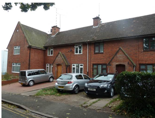
Hedges removed at the front of properties on Chantry Place to provide access for cars and use of white UPVC window frames
