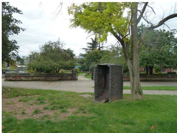
Redundant brick structure that intrudes on views of the north entrance space near the north entrance to the gardens
