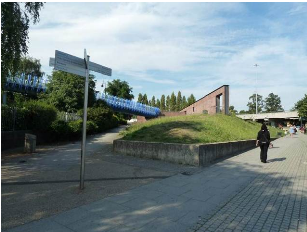
Worn areas of grass on the mound at the entrance to the garden from Hales Street
