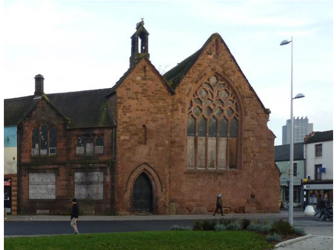
Timber sheets covering windows of the Old Grammar School.
