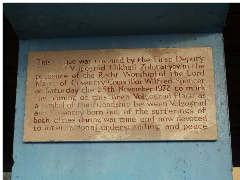
Commemorative plaque in need of refurbishment
