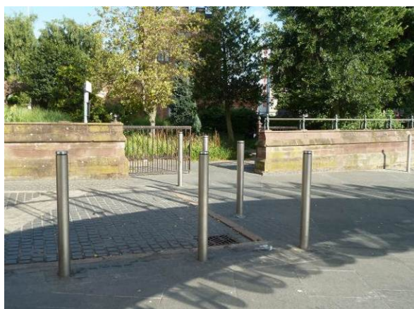
Bollards adjacent to boundary wall of Lady Herbert's Garden
