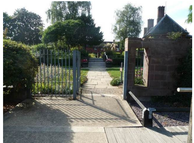
Galvanised steel fence and gate
