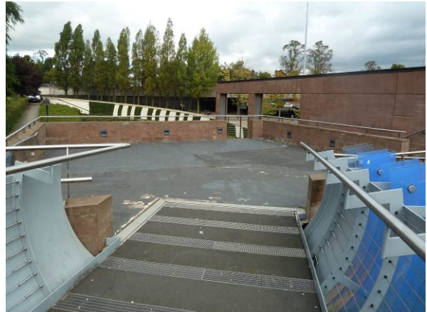
Lack of signage at entrance to garden from the glass bridge
