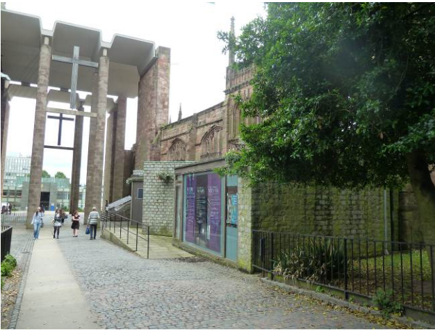
The book shop which abuts the north side of the Cathedral ruins and whose overall design and use of materials does not complement the historic building
