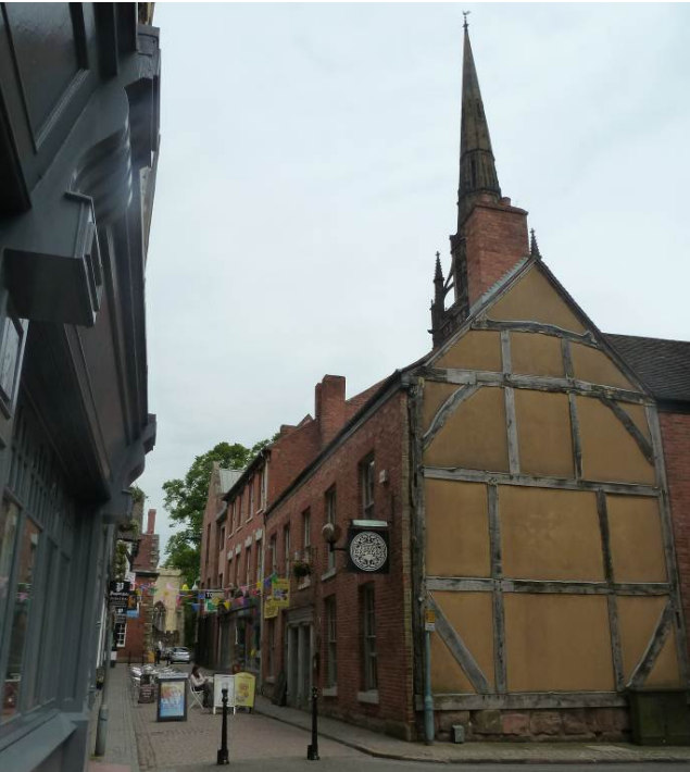
View along Hay Lane from High Street
