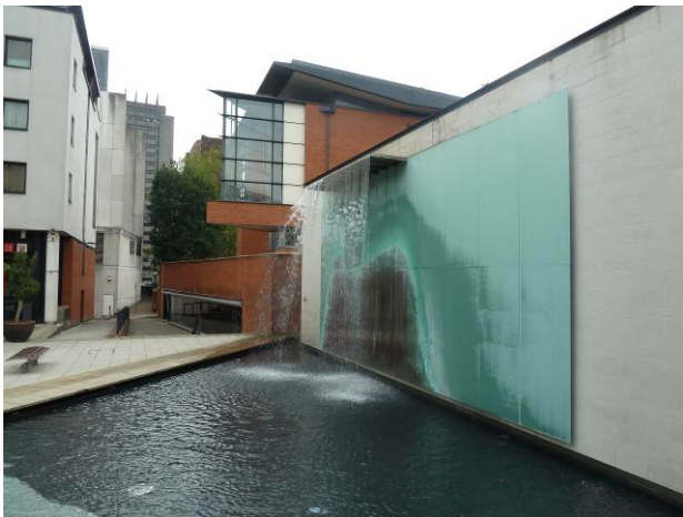
Waterwindow installation from Priory Place (above) and from the Cloister Garden (right)
