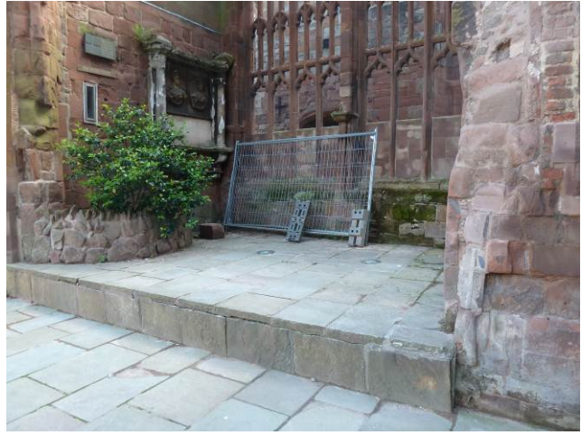
Redundant barriers left in Cathedral ruins
