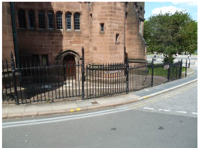
Railings style at south east corner of the old cathedral in keeping with the historic building
