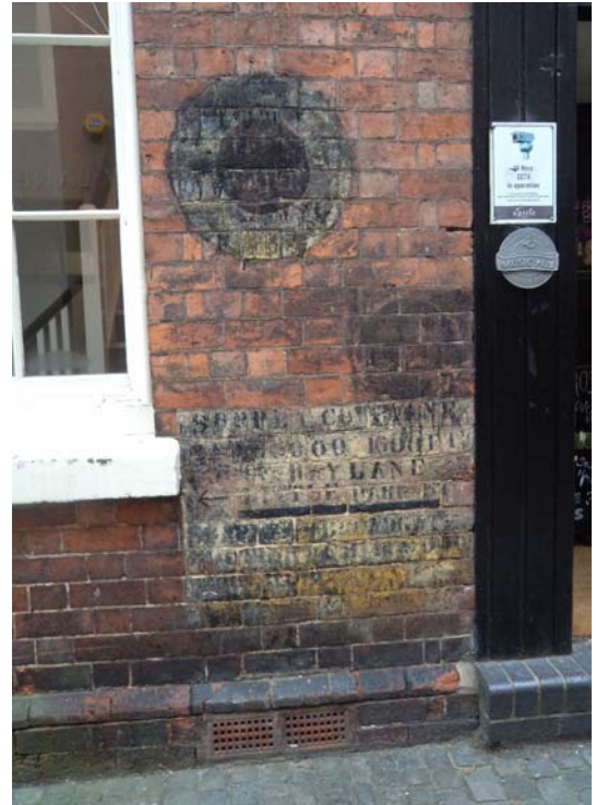
Second World War painted water supply signs giving instructions to blitz fire-fighters
