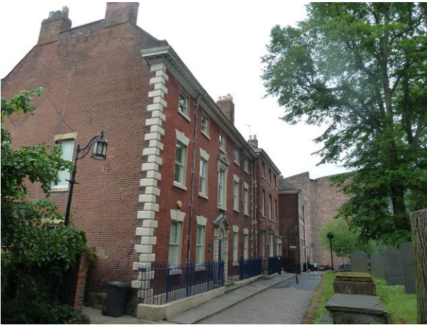
Pelham Lee House, Priory Row
