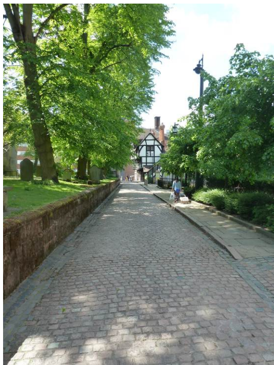
Cobbled street surface on Priory Row
