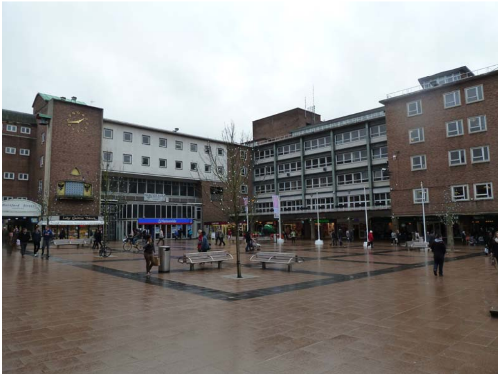
Grade II Listed Broadgate House, Broadgate
