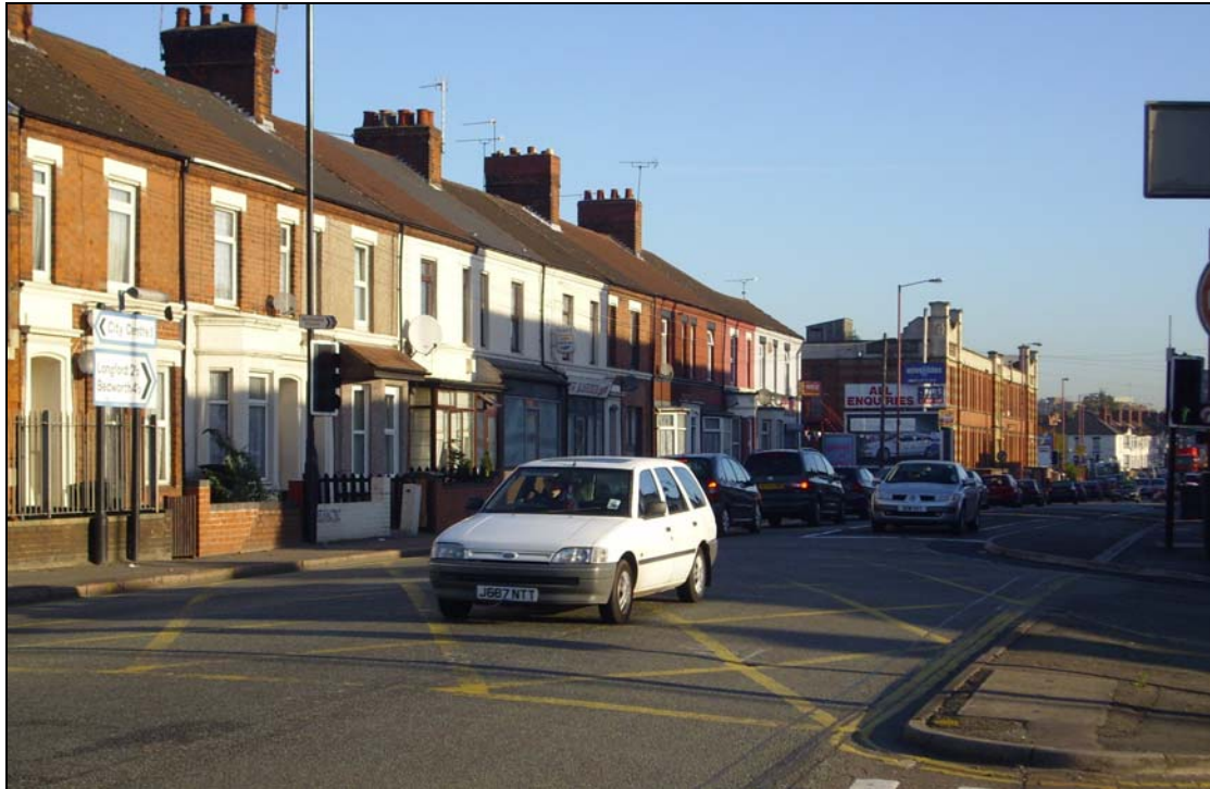
Figure 5: Foleshill Road at Junction with Eagle Street
