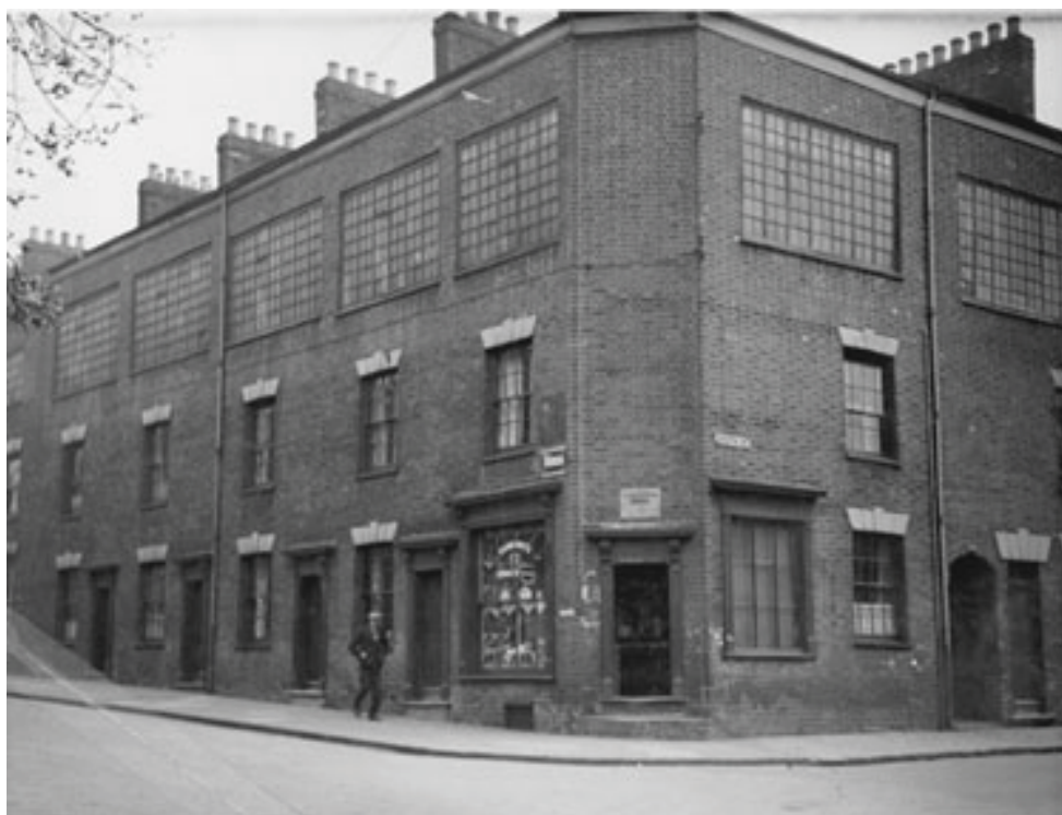
Three-storey ribbon weaving top shops in South Street (Reproduced by permission of Coventry History Centre, Herbert Museum and Art Gallery)
