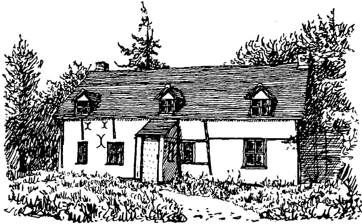
Dormer Cottage, Washbrook Lane Render, half timber, plain tiles and dormer windows
