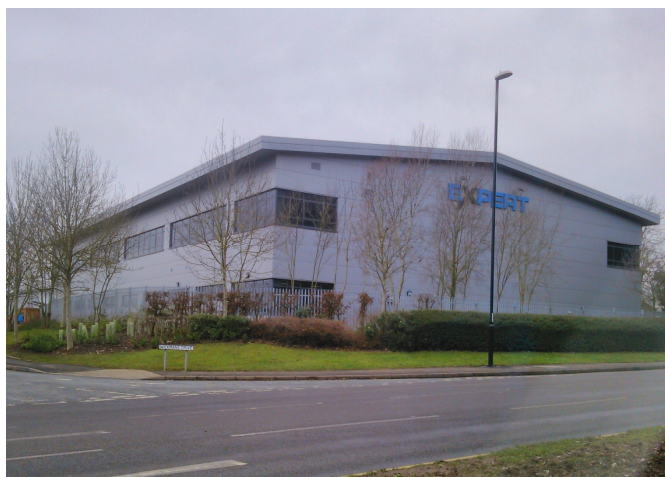
Picture: Completed manufacturing unit at Wickmans Drive.
