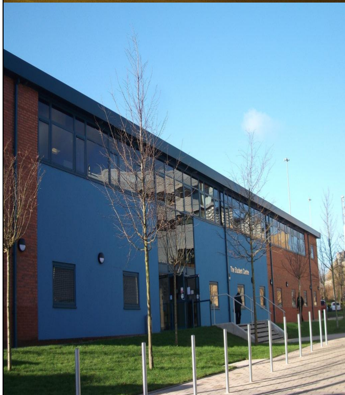
Severn Trent Offices and Car Park
