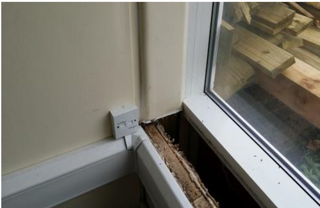
AIB panels beneath windows – AIB panel exposed below window board
