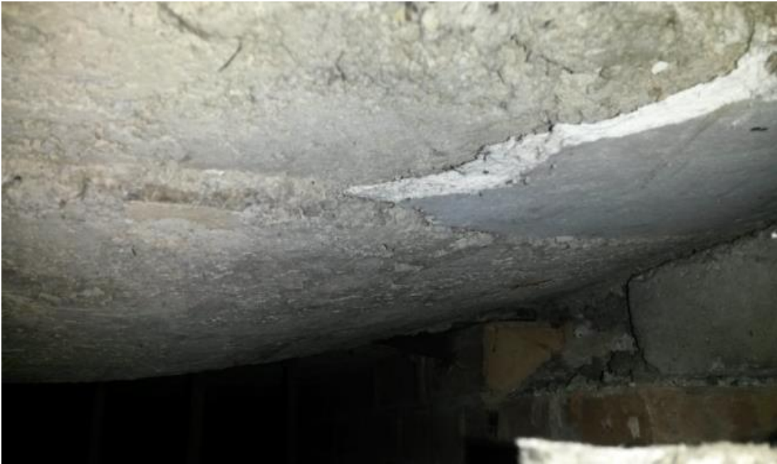
Sub floor heating ducts – insulation board shuttering around duct hatches
