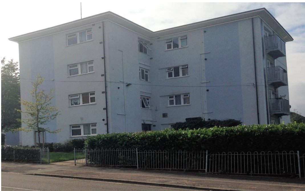
Refurbished flats on Robin Hood Avenue
