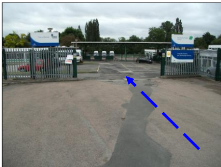
Photograph 2: Run-off drains into school parking area. School entrance has no surface water resilience.
