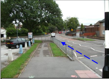
Photograph 4: Water accumulates downstream end at main school access.
