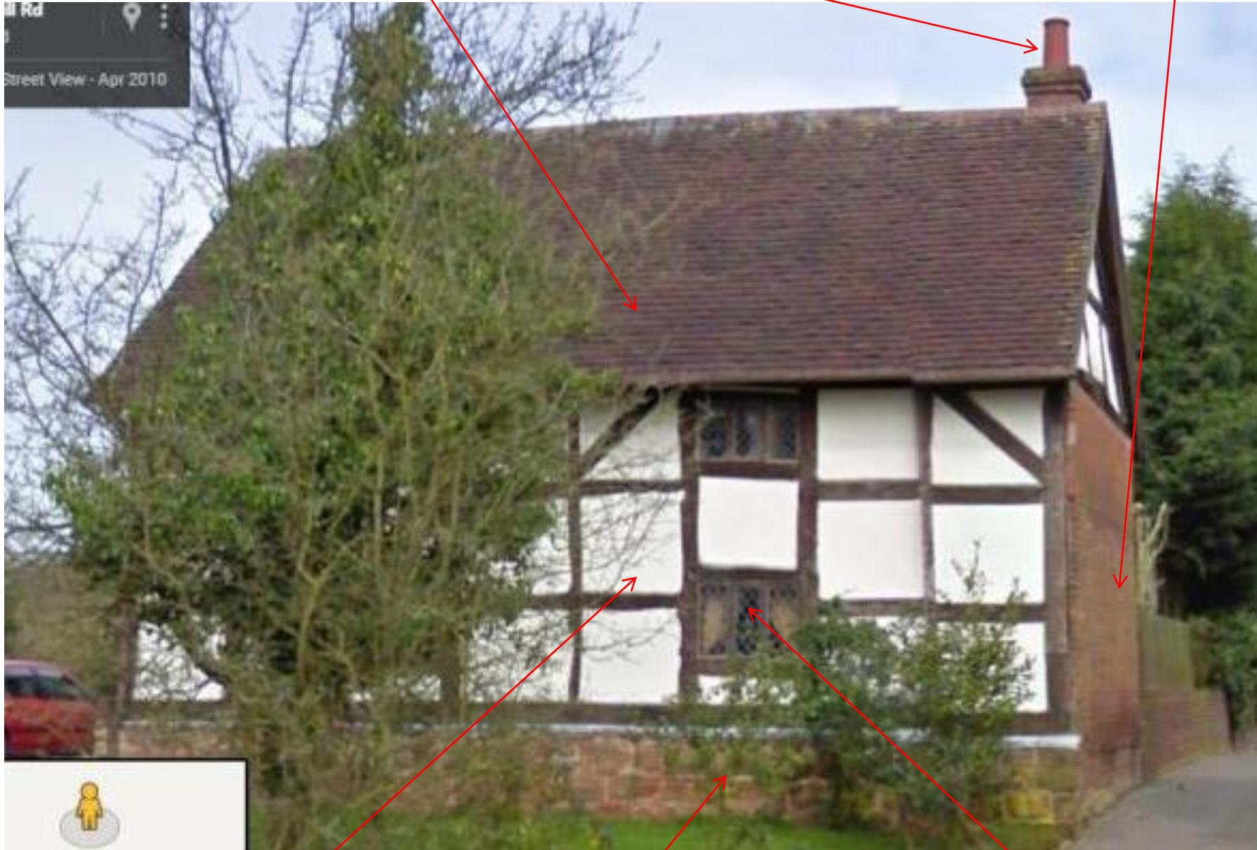
Timber frame with infill panel construction
