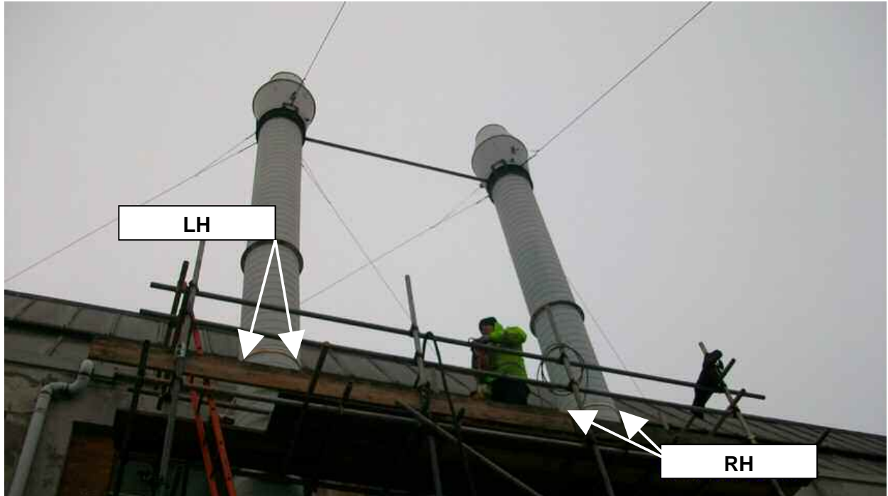
Schematic Photograph Industrial Spray Booth 1 Emission Points LH & RH.
