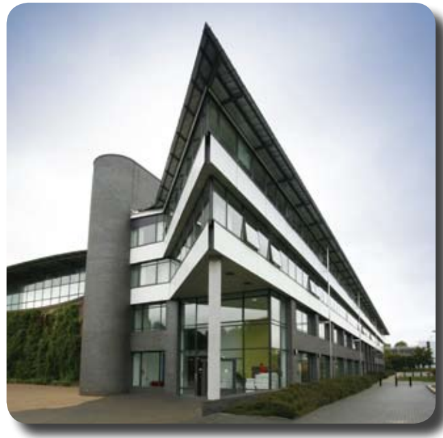
Warwick Manufacturing Centre
