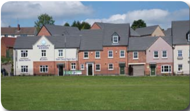
Camp Hill regeneration scheme, Nuneaton
