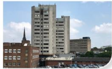
City Centre South Demolition of Coventry Point
