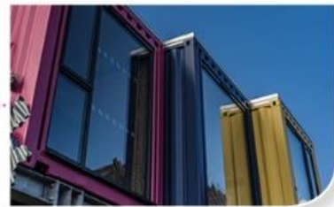
The Box at FarGo Multi-purpose events space
