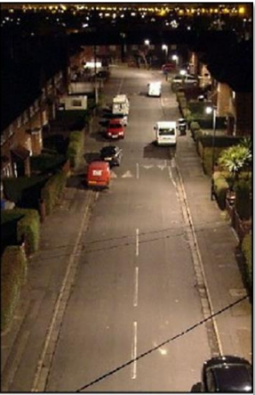
New Street Lighting
