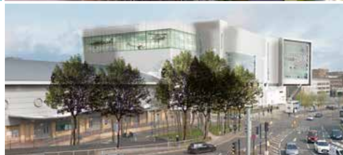
Pictured: Above, battery production could start at Coventry Airport in 2025. Below, IKEA building set to store nation's arts treasures.
