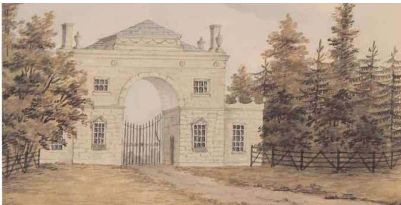
Coombe Abbey West Lodge. The principal entrance to Brown's Parkland.
