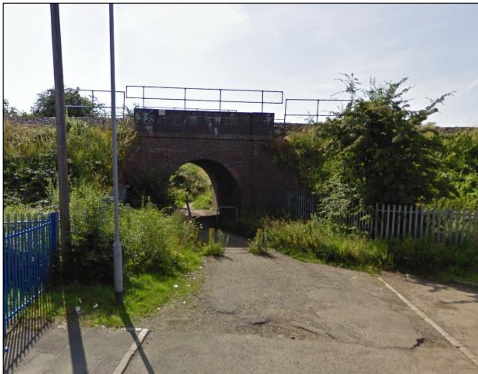
Figure 6-7 - Existing railway bridge north of Blackhorse Rd (Extracted from Google Streetview 2019)
