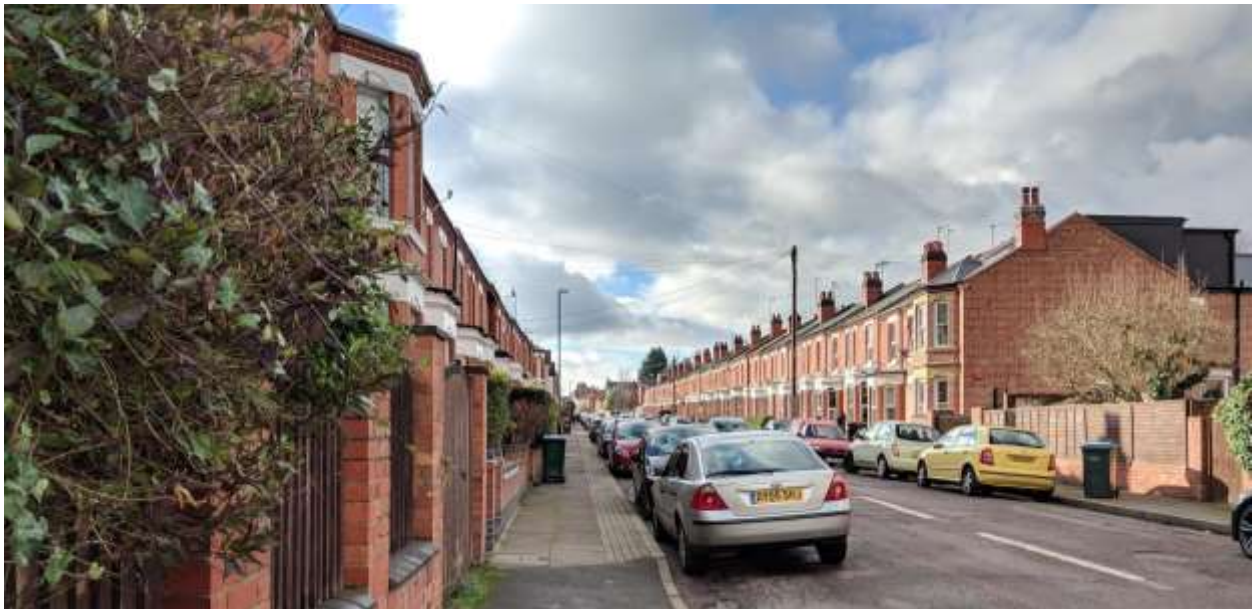
Fig 3.27. Berkeley Road North is characterised by significant groups of red brick terraces (with some examples of roughcast render) incorporating stone banding and hoods around windows and doors some of which incorporate a pattern, as well as key features such as chimneys which provide a strong rhythm to the road. Despite a strong terrace rhythm many historic windows have been lost, boundaries rebuilt and at least one example of a red brick facade being inappropriately rendered.
