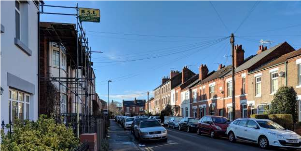
Fig 3.7. Berkeley Road South is a mix of terraces at varying scales, incorporating some semi-detached dwellings. These include larger-scale terraces with historic top light windows. Detailing includes decorative brick patterning to the eaves, stone window and door hoods, and chimneys.
