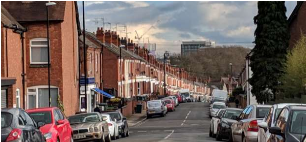
Fig 3.19. Newcombe Road provides views back to the City Centre. Despite a strong terrace rhythm with a run of smaller-scale red brick terraces incorporating chimneys and stone detailing enhanced by a curving street structure, the group has been undermined by visual clutter including satellite dishes, tv aerials, bins, as well as alterations to windows and front boundary treatments.
