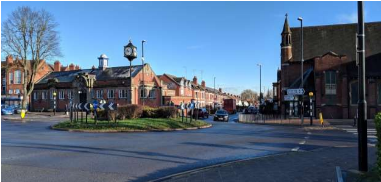
Fig 3.17 The junction of Earlsdon Street, Earlsdon Avenue South, and Poplar Road, marked by the central clock, straddles three localities, and provides a significant nodal point and gateway in the area. The significant grouping of the clock, Earlsdon Methodist Church and Earlsdon library provide an important focal point at the gateway into the Newcombe Road locality.
