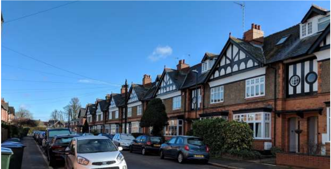
Fig 3.14. To the east side (right) of Avondale Road there is a terrace with a highly significant surviving decorative pattern incorporating half-timbered gables topped with roof finials, chimneys, bay windows, a contrast between brick and roughcast render (separated by brick banding) and round oculi windows. Whilst the terrace is enhanced by front boundary soft landscaping, there has been loss of historic boundary treatments and hard-standing/surface materials.
