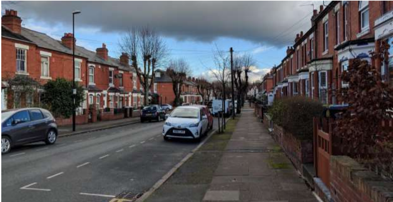
traditional sash windows remain, many have been replaced with uPVC top hung windows and traditional boundary treatments have been rebuilt.
