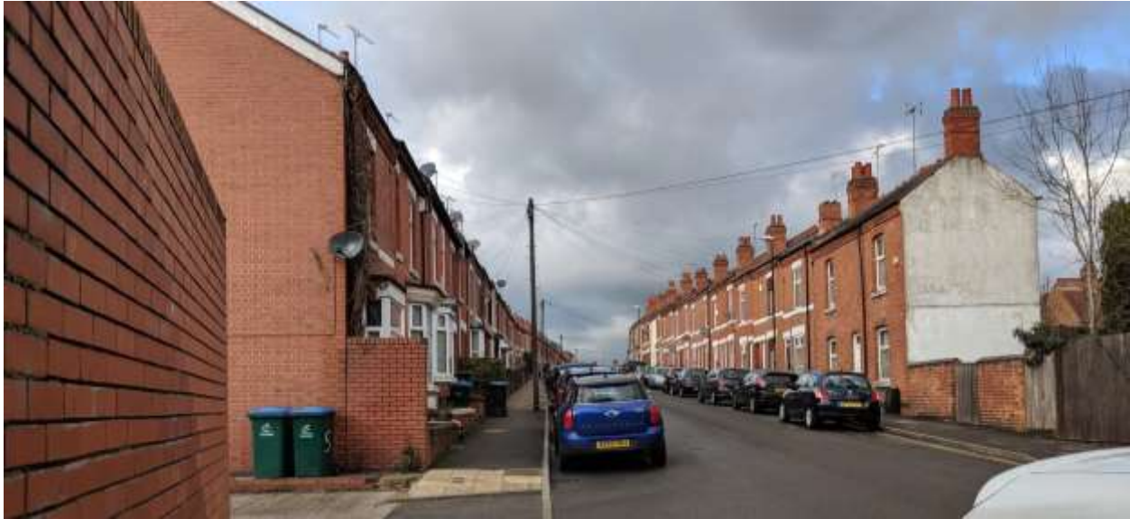
Fig 3.20. Poplar Road is characterised by a strong terrace rhythm, formed from smaller-scale red brick dwellings. These incorporate stone detailing around windows and doors, as well as brick patterning to eaves level. Despite this strong rhythm, the group value of the terrace has been undermined by the loss of historic boundary treatments, intermittent rendering of historic red brick houses, and general visual clutter including satellite dishes, as well as loss of historic windows.
