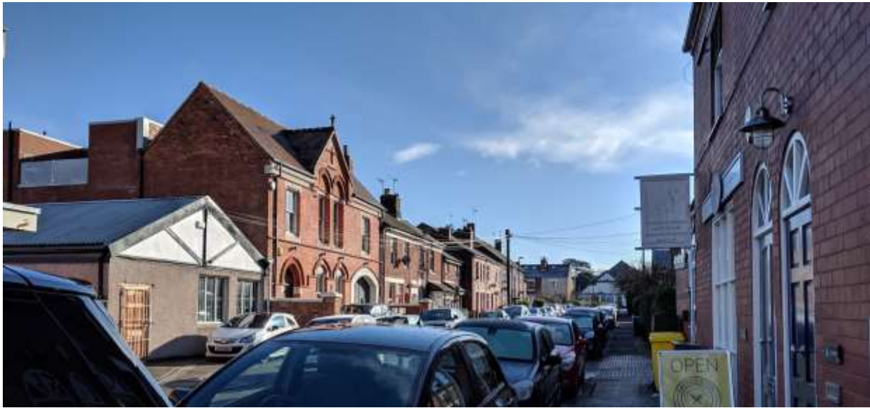
Fig 3.6. Moor Street incorporates a former nail factory, now converted to offices, alongside a series of terraces with some later infill. Key losses along this road include historic boundary treatments (rebuilt), and windows. At least one brick terrace has been inappropriately rendered. The Criterion Theatre, provides an important visual terminus to the road.
