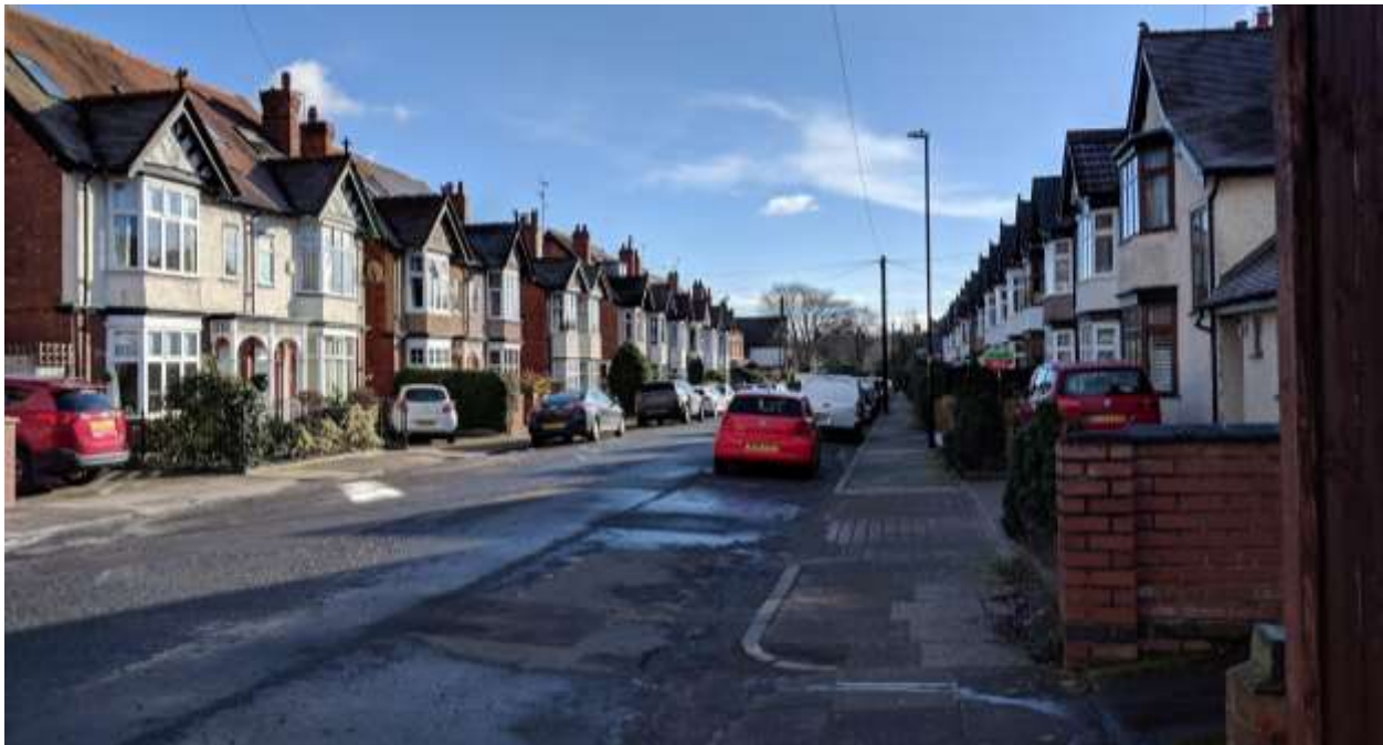
Fig 3.12. Shaftesbury Road is characterised by a surviving group of semi-detached brick and rendered dwellings, in a strong building line with a series of half timbered gables topped with roof finials. Some of these incorporate historic timber porches. There has been an evident loss of historic boundary treatments along this road.
