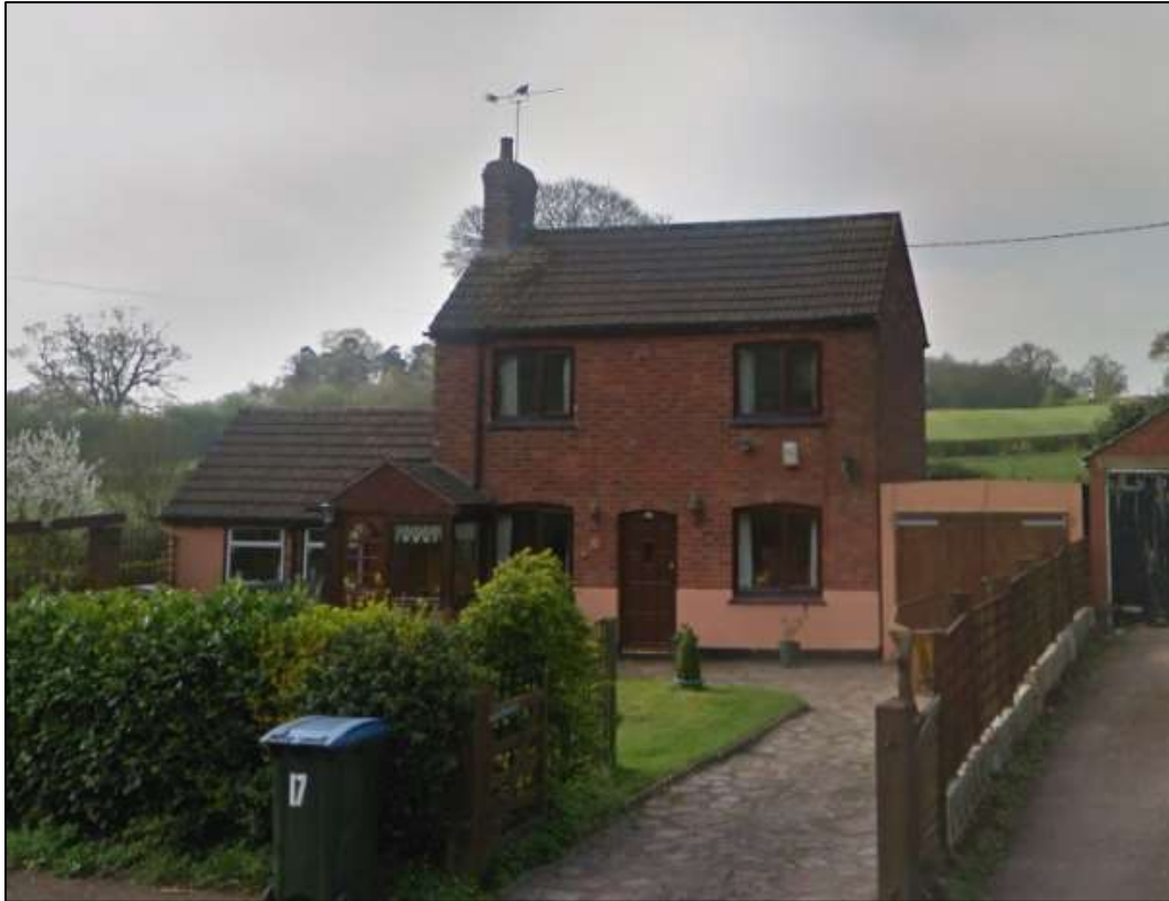
Figure 7: 17 Wall Hill Road
