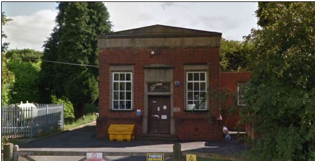
Figure 14: Locally Listed Pumping Station
