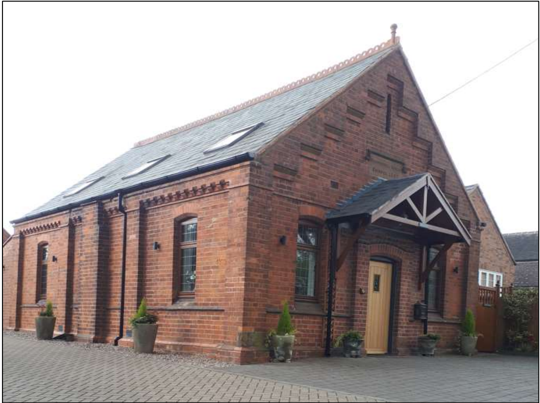
Figure 20: Locally Listed United Reformed Church, Hawkes Mill Lane.
