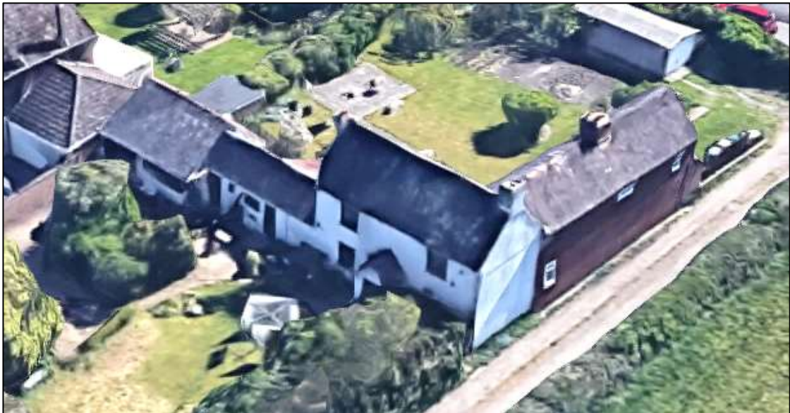
Figure 9: 29, 31 & 33 Wall Hill Road
