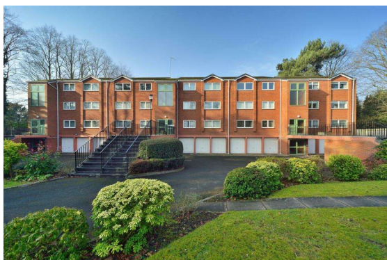
Figure 8.6 – Mount Gardens Building
