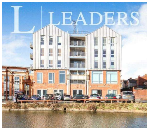
Figure 8.9 – Boiler House Building
