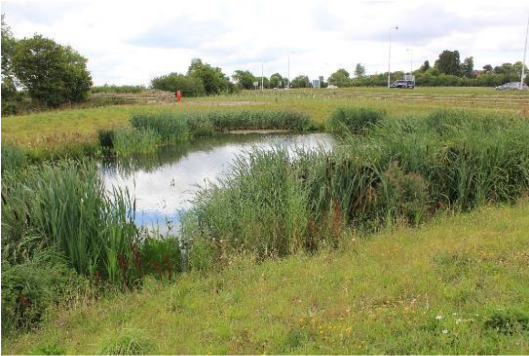
Sustainable drainage for road improvement scheme near Gaydon.
