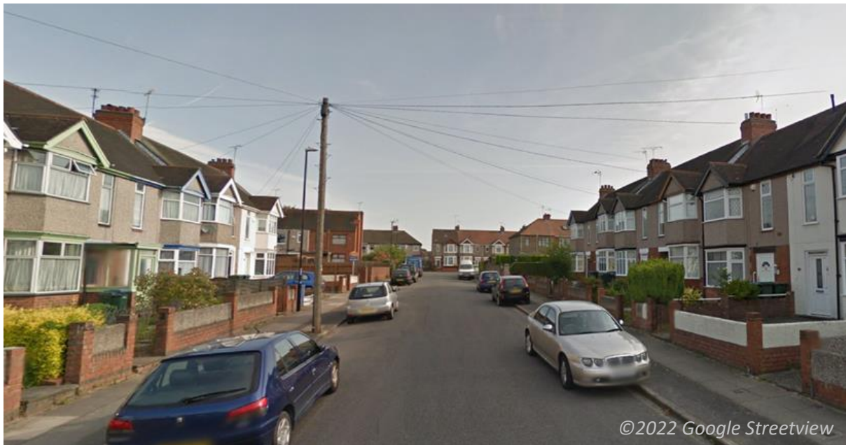
Figure 16: Images showing i) two story suburban residential accommodation and ii, iii) taller residential development in the city center.
