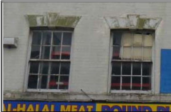
Sash Windows to Number 93
