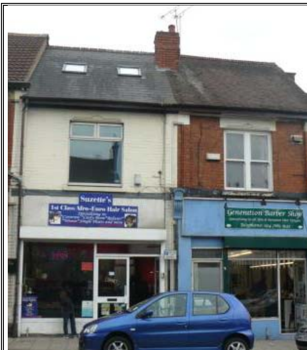
Rooflights and Wiring
