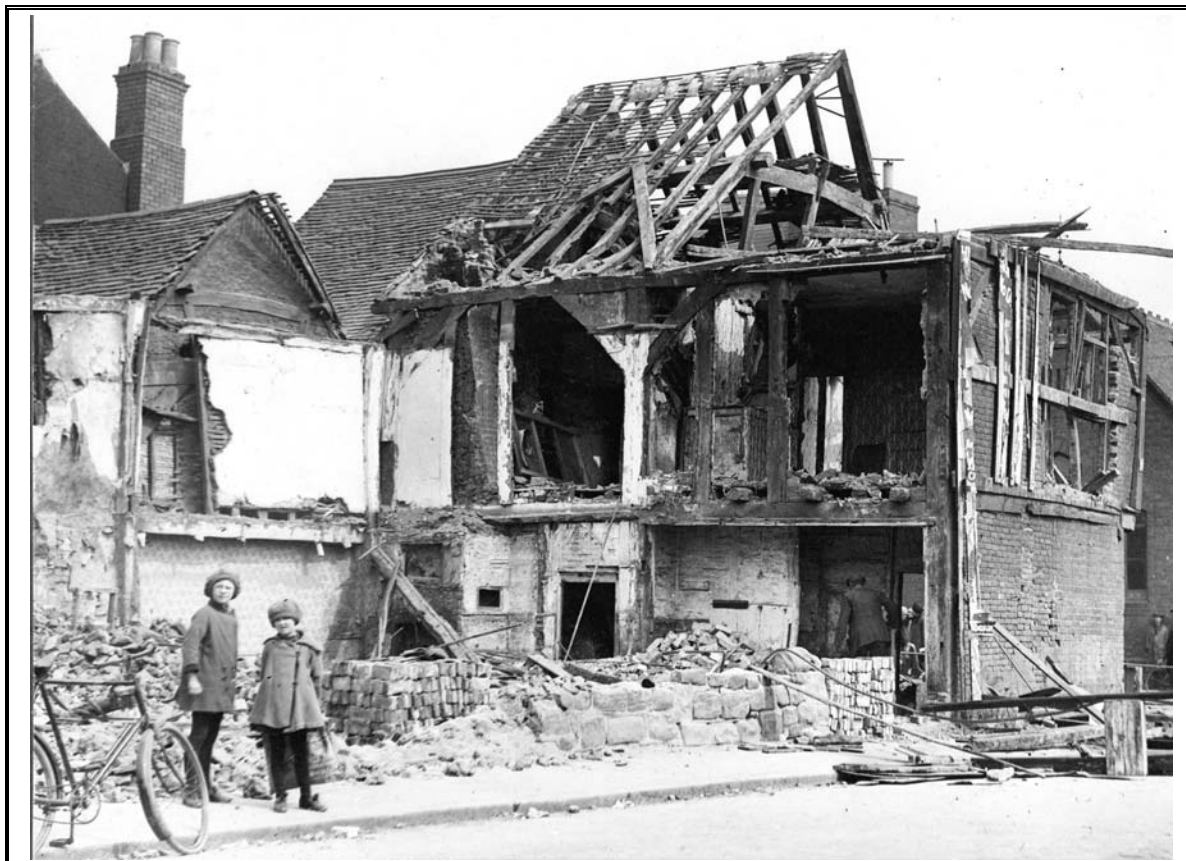
Demolition of Nos. 26 and 27 Far Gosford Street
