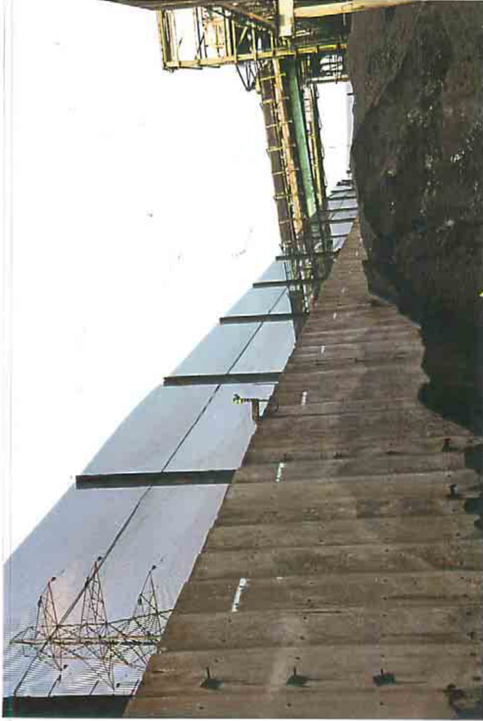
Stocking Enclosure Environmental control measures in place; wind break mesh water sprays and height marks on the stelcon walls.
